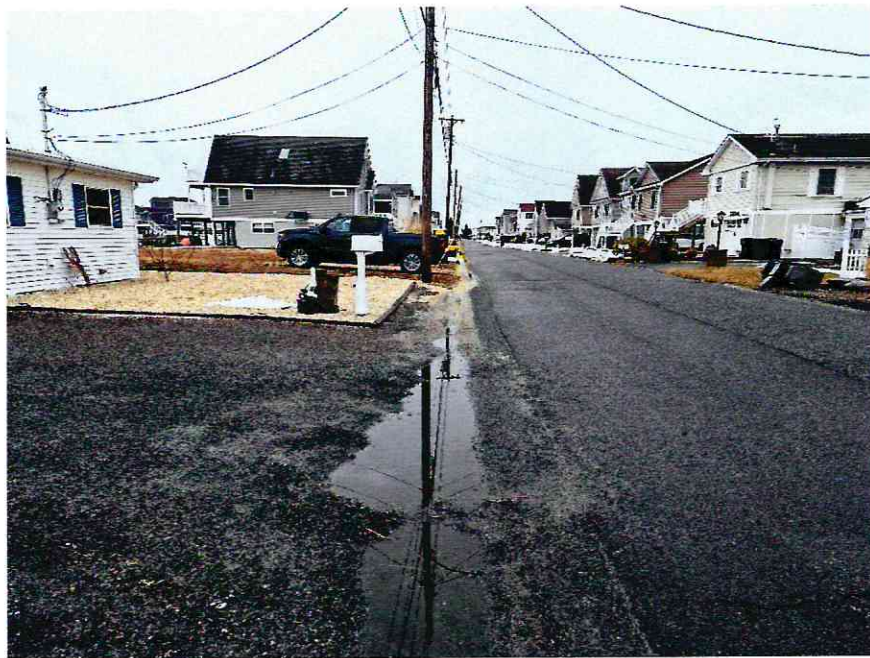
View of East Sail Drive looking in an easterly direction.
